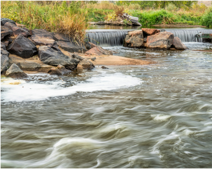
Water diversion dam on the South Platte River in northern Colorado below Denver.
