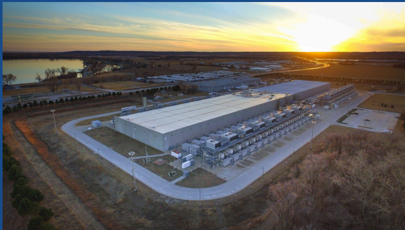
Aerial view of the Google Data Center in Council Bluffs, IA.
